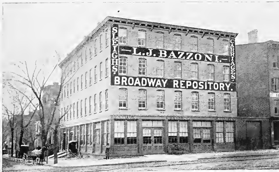
BAZZONI BUILDING—Corner of Grand Street and Broadway
